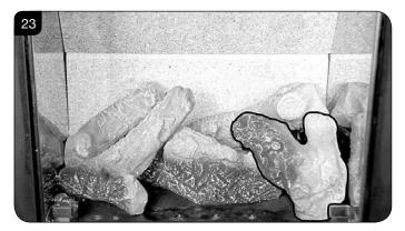
9.8 Use some of the Embaglow provided and cover the ports in the burner tray with a liberal amount of fibres. Use a small piece in front of the log on the left hand side and a long strip in front of log B, see Diagram 24.
