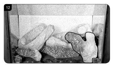
7.8 Use some of the Embaglow provided and cover the ports in the burner tray with a liberal amount of fibres. Use a small piece in front of the log on the left hand side and a long strip in front of log B, see Diagram 13.
